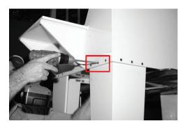
2. Mount the pump motor. Use a 7/16" wrench to attach/mount the pump under the shelf on the right side of the booth, holes (bolts and nuts are provided).
